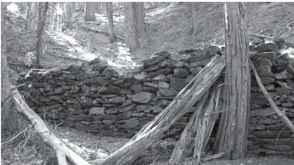
Hand-staked rock wall along an old wagon road at the Heath Mine, Argentine, 2008.
