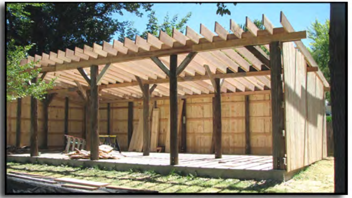
Museum's new pole barn well under way last summer.
