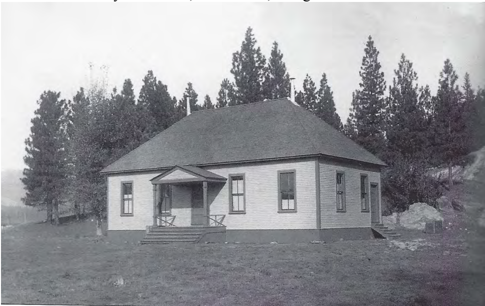
Temporary Plumas County High School, near the base of China Rock.
