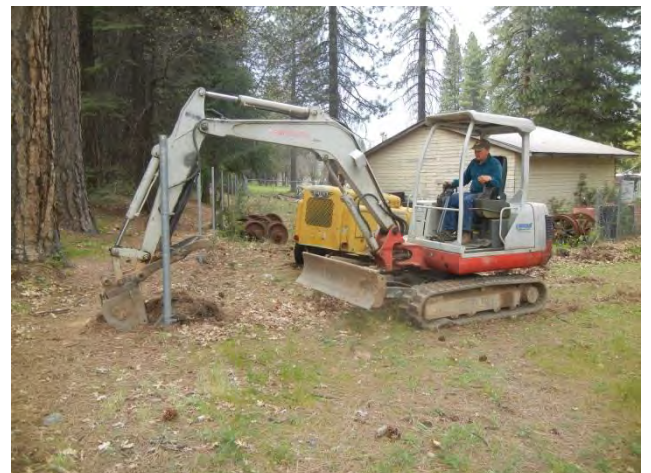
Norman Lambert clearing the way for rebuilding a fence along the Spanish Peak Locomotive track.
