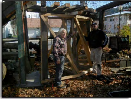
Rich Knoettgen, chief engineer and designer of the stamp mill-ore car trestle, and his helper Jim Boland are close to finishing this stupendous project.
