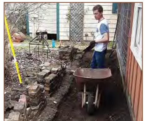
Sam Lawson digging out bricks.
