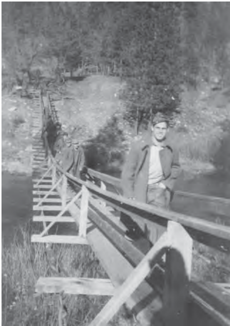
“Thomas and gang returning to work after lunch on suspension bridge over East Branch of North Fork Feather River, January 1934.”
